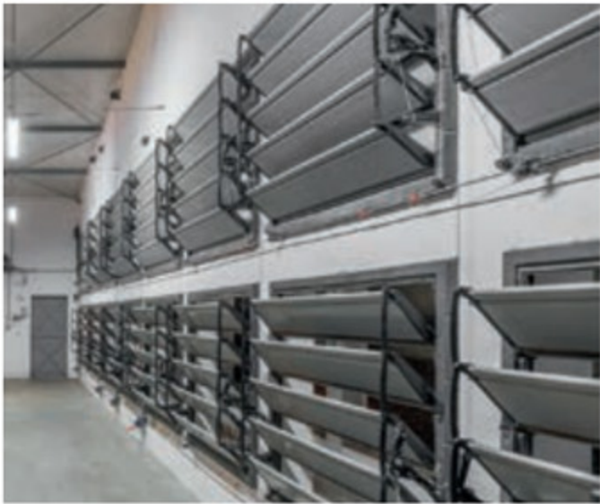
MultiVent 17 M in the gable wall for tunnel ventilation
