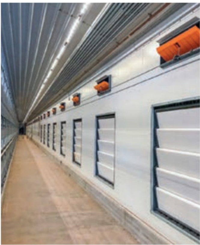
Aviary house with CombiTunnel ventilation, using CL 1911 F wall inlets and MVT shutters
