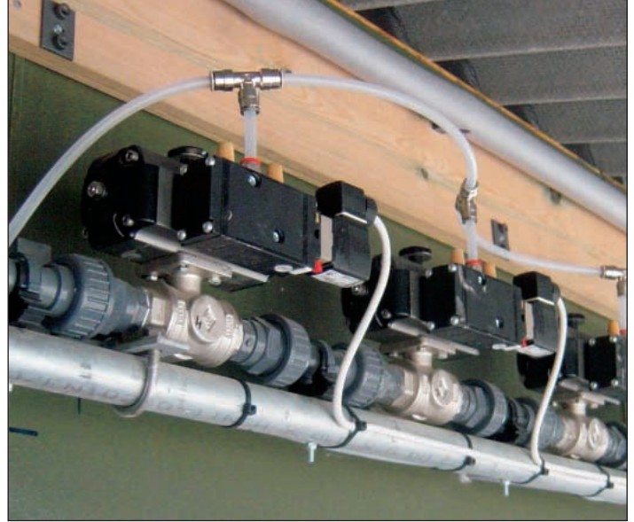
Installation of feed valves in the central passage
